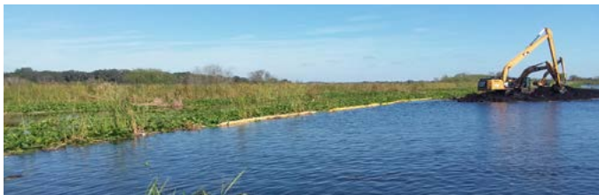
In cooperation with SJRWMD, FWC has worked to breach the levees that divided the Emeraldalda Marsh system from Lake Griffin.
